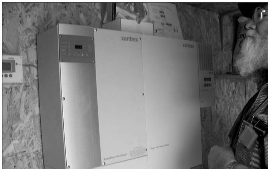
The inverter that converts the DC output to AC output is shown to the left. The inverter puts the power into a form that can be used in your home.
